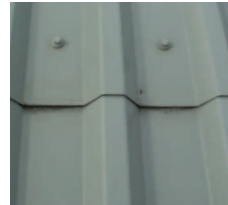
Colorcoat HPS200™ with Galvalloy™ roof after 7 years.
